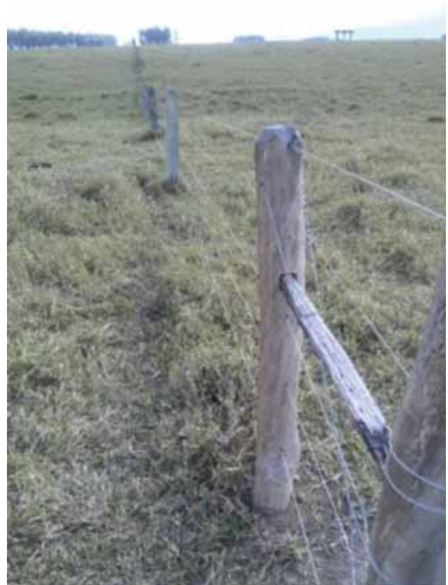
Figure 1: Wire fence constructions are very often cadastral boundaries. Those fences can be easily detected with radar.
